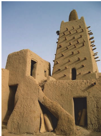
Figure 1. Objects implemented technique is traditionally raw earth: the city of Timbuktu in Mali in Africa
