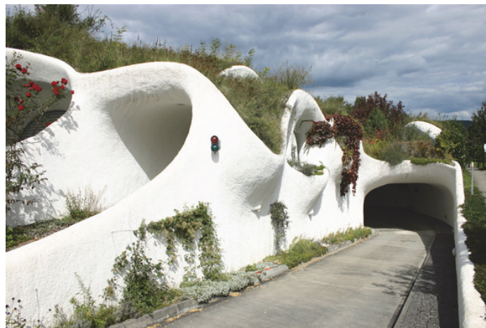
Figure 2. Facilities technique of raw earth and shotcrete: Earth House Estate Lättenstrasse, Dätikon, Switzerland
