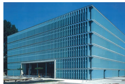
Figure 1 - EMPA zero energy office
