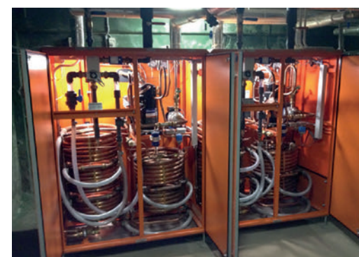
Figure 5 - Wastewater heat recovery system (Gazette “REA vēstnesis” 2014)
