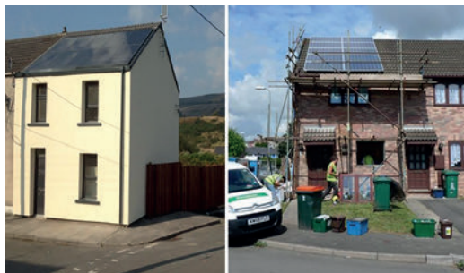
Figure 3 - Examples of social housing retrofit. Figure 3a shows a recent retrofit where the whole south facing roof has been replaced by a PV panel. Figure 3b shows a 'bolt on' approach to PV
