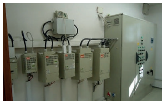
Figure 10 - Monitoring operating systems
