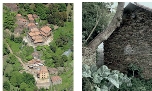
Figure 1 - Left - Aerial view of a vernacular settlement in the central region of Portugal. All houses present massive masonry exterior walls of shale stone and the structure of the roofs in natural timber.
