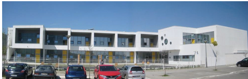
Figure 1: Kindergarten "Tesla – Science for Life" in Block 67, New Belgrade. Design: DVA STUDIO. Photo: D. Vasović.
