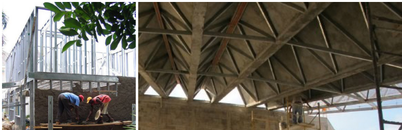
Figure 5. Construction of building in Am-cor system.
