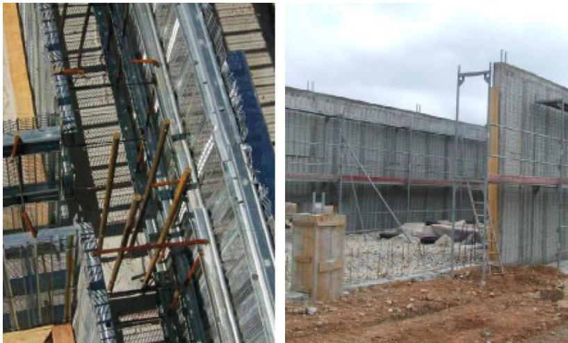
Figure 7. The system of integrated metal formwork.
