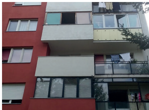
Figure 4 - Building appearance after refurbishment, street Dr. Nike Miljanica, Karaburma, Belgrade
