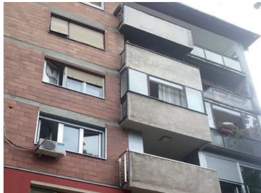
Figure 3 - Building appearance before refurbishment, street Dr. Nike Miljanica, Karaburma, Belgrade
