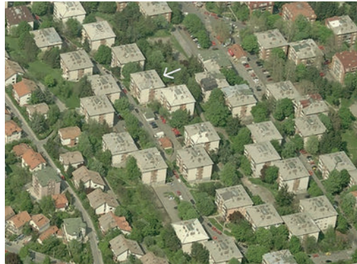
Figure 2 - Position of the retrofitted building on the street, Dr. Nike Miljanica, Karaburma, Belgrade
