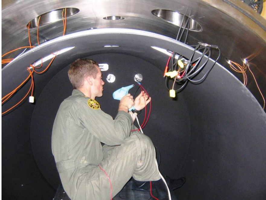
Figure 29: AFIT TVAC Power Lines Installation.
