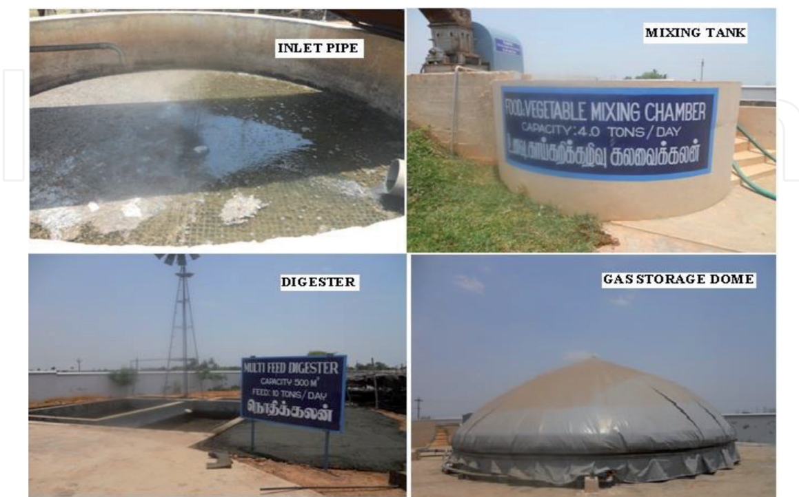
Figure 12. Biomethanation process.
