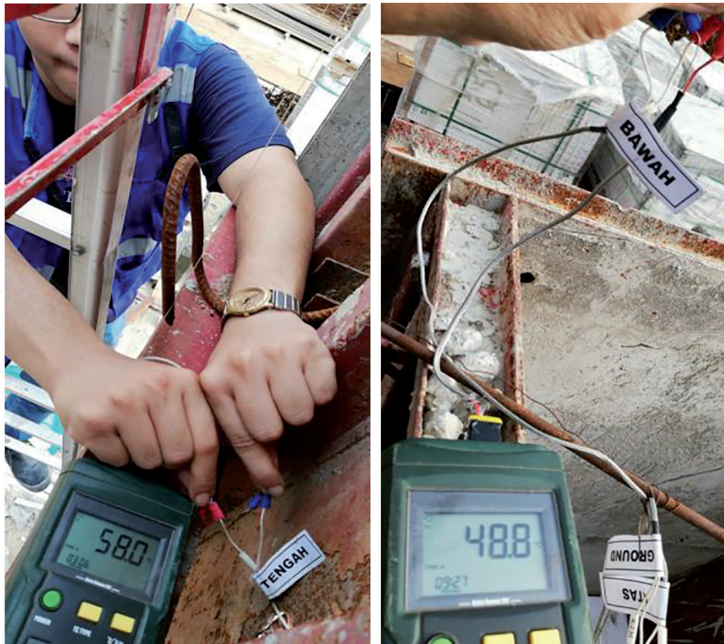
Figure 18. Bioconc LHC mock up thermocouple monitoring.
