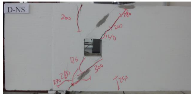
(c) close view of the crack pattern
