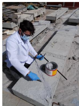
(b) Epoxy filling
