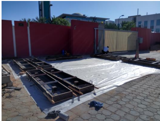
(a) Casting area
