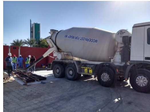
(b) Ready-mix concrete
