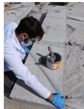
(c) CFRP strip insertion
