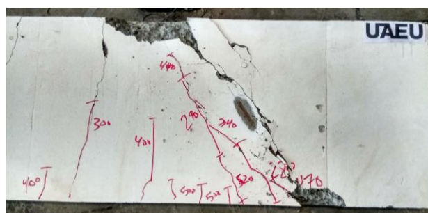
(c) close view of the crack pattern
