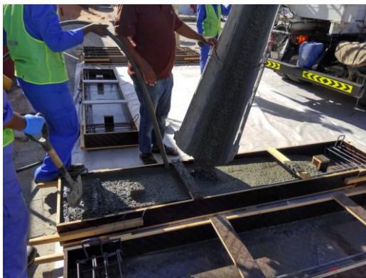
(c) Concrete pouring and vibration
