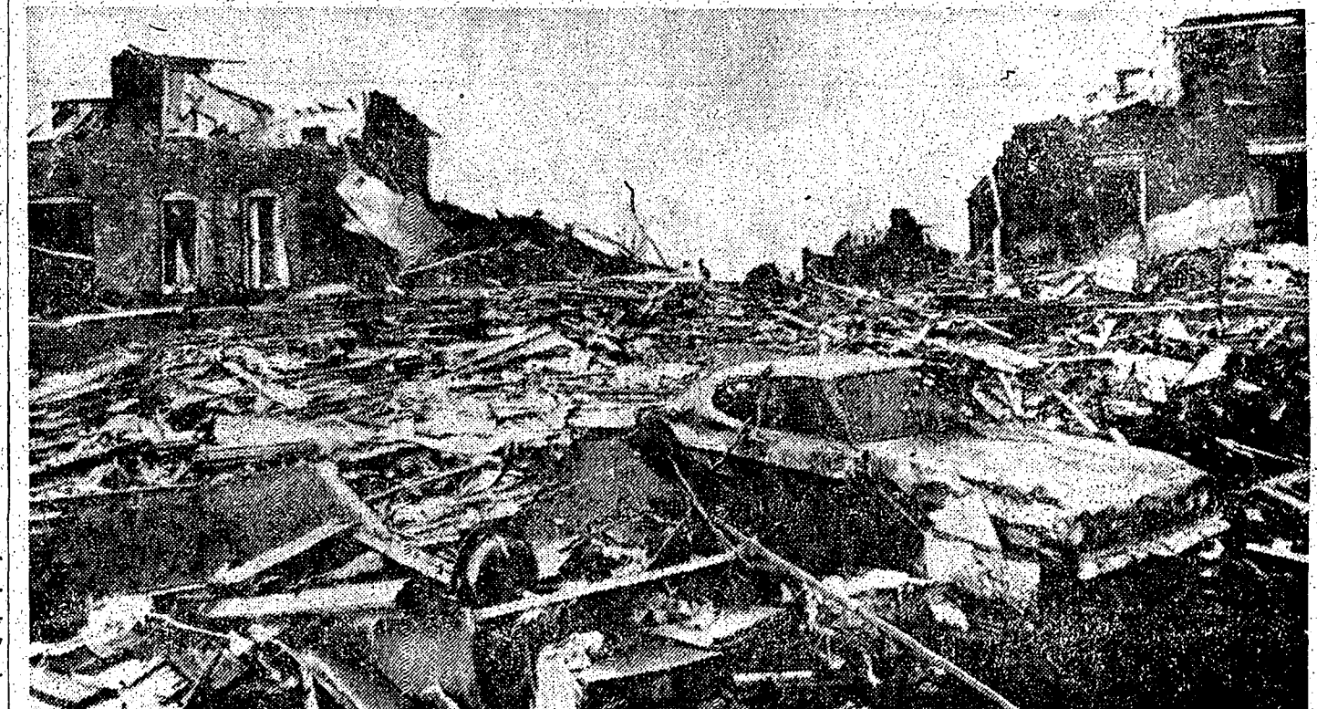
RAVAGED HOMES . . . Debris litters the streets in the city of Northfield in Louisville's eastern suburbs after a tornado ripped through eastern Jefferson County. Five persons were reported dead in Jefferson County and as many as 36 in Kentucky as a whole. Tornadoes ravaged much of the Midwest Wednesday. (AP Photofax)
