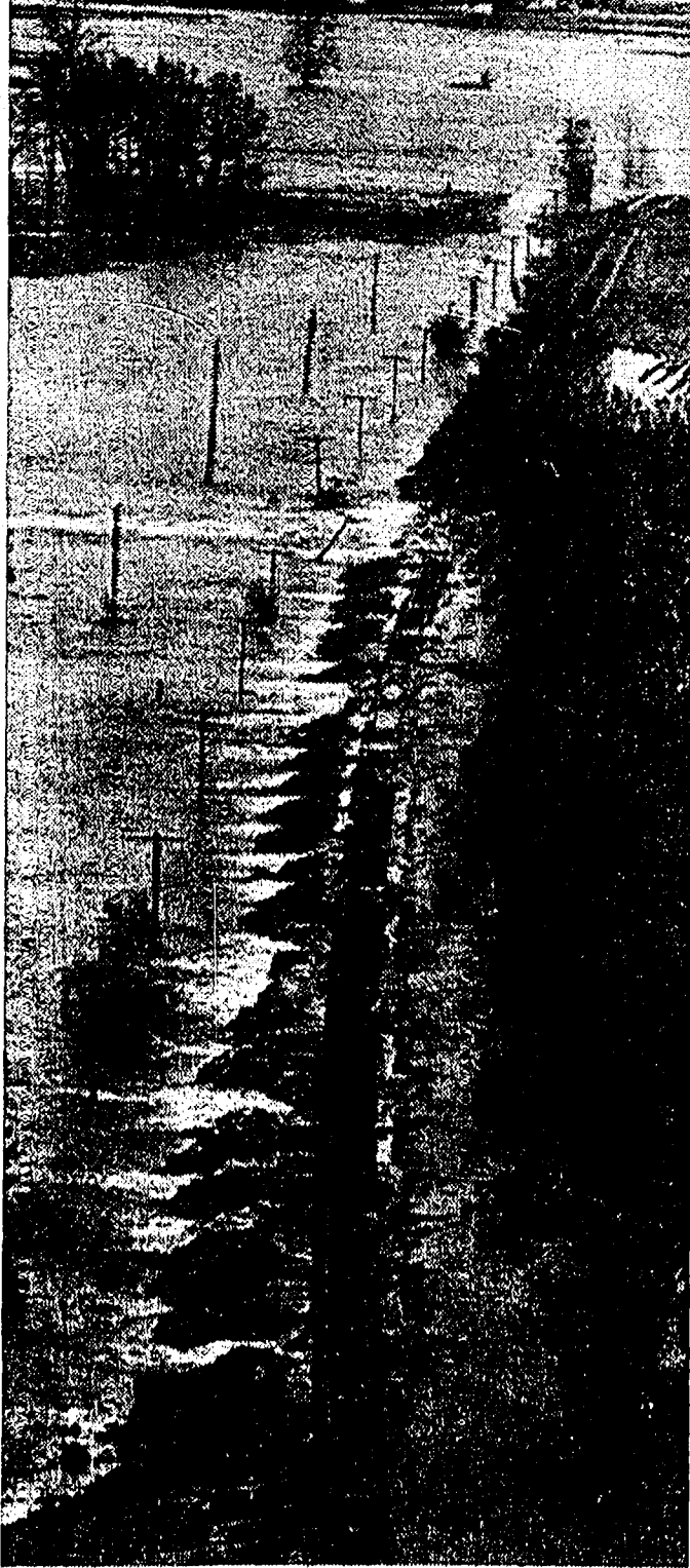
WASHOUT . . . Flood waters of the Missouri river wash over a railroad levee in St. Charles, Mo. The washover caused about 600 people to evacuate their homes in the St. Charles area. (AP Photofax)
