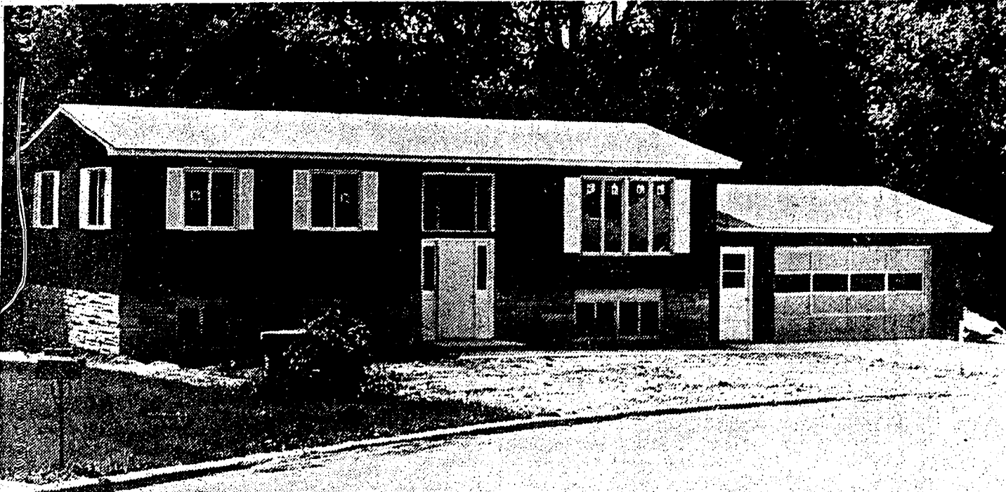
RANGE OF PRICES . . . Starting price of the homes is $12,650. Two basic home styles, ranch-type and a split-foyer, are available in a wide range of variations. The initial concept of the modular home idea was to enable persons to own their home at a reduced cost.
