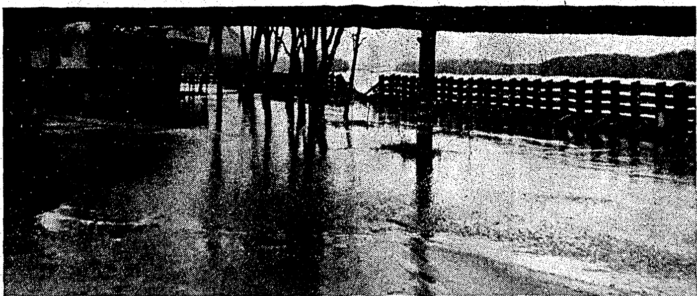
DAMAGED RETAINING WALL . . . Only remaining evidence of a Sunday accident on the Mississippi River, involving a towboat and four barges, at the Chicago-Milwaukee Railroad's swinging Mississippi River bridge, right off Shore Acres, near La Crescent, Minn., is the above damaged wooden retaining wall. The four barges being towed by the Hortense B. Ingram, two loaded with petroleum and two empty, slammed sideways into the railroad when carried by the strong
