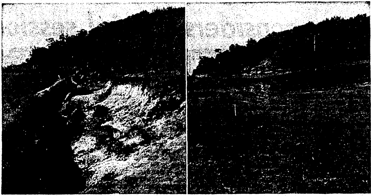
PROBLEM SOLVED . . . At left is a problem, a badly eroded drainway. The gully gets deeper every time rainfall and runoff occurs. At right, the same scene five months later after a soil conservation grassed waterway treatment. The gully was filled, a flat bottom constructed and it was seeded and fertilized, controlling erosion and sediment. The former gully can be utilized for hay. (Olin Fimreite photos)
