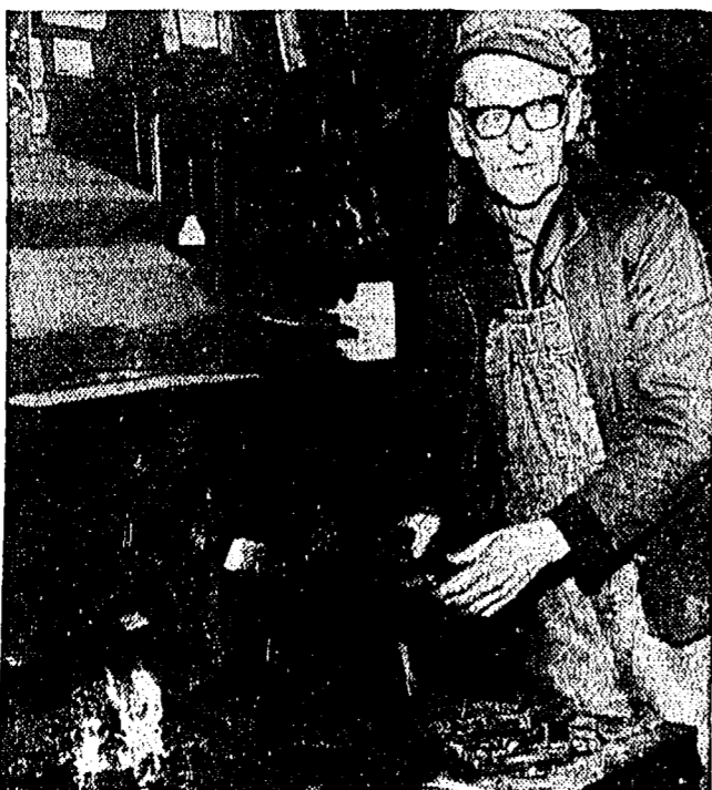
FORGING IRON . . . Mike Tibor says a special coal, the correct degree of heat and a clean fire are needed to forge iron.
