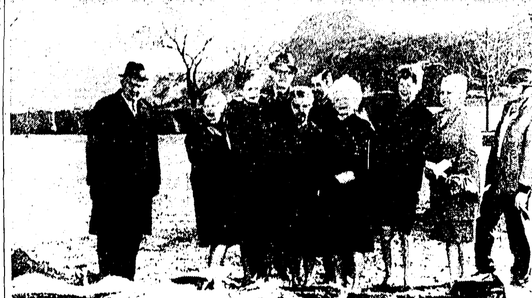
GAZEBO CONSTRUCTION BEGINS . . . The Soroptimist Club has donated $2,000 to erect a gazebo near the Rose Gardens in Lake Park. Members shown viewing the construction site are, from left: Mayor Norman Indall, Miss Harriet Kelley, Mrs. Marie Pj-
