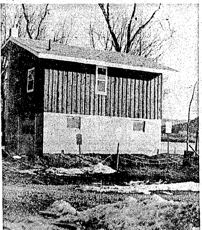
TO KEEP IT OFF THE FLOOR . . . The cottages of Lester Senty, Independence; Dr. Elmer Rohde, Galesville, and Ed Kiedrowski, bordering the Mississippi River have been raised more than seven feet to escape a possible flood.
