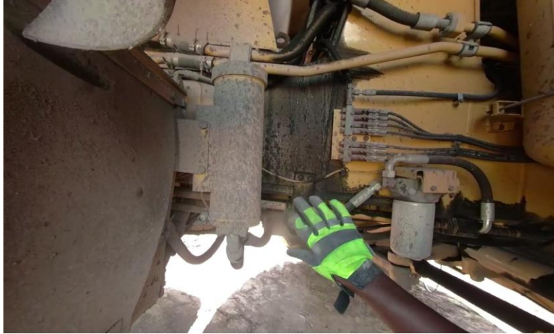
Figure 36 - 360-degree Video – Inspection of Hoses
