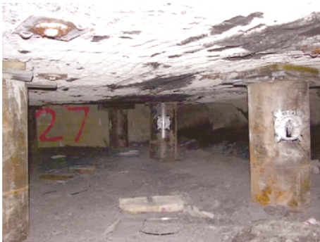
Fig. 1. Installed The CAN® roof supports in mine entry, 0.46 m diameter.
