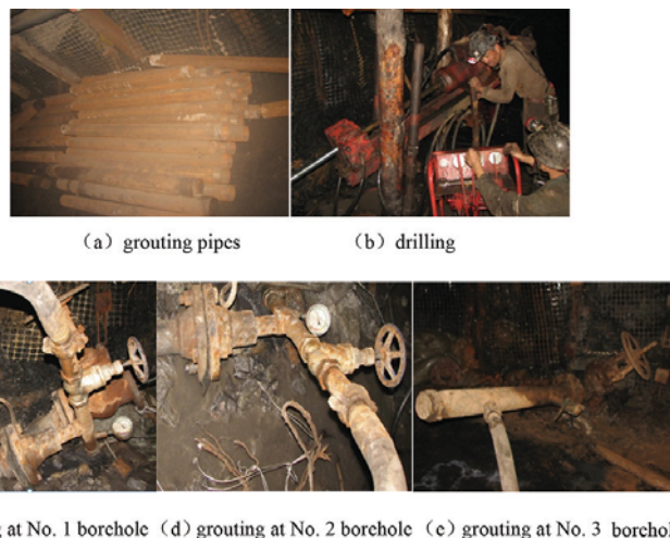
Figure 10—Grouting borehole drilling and grouting at Dongjiahe coal mine
