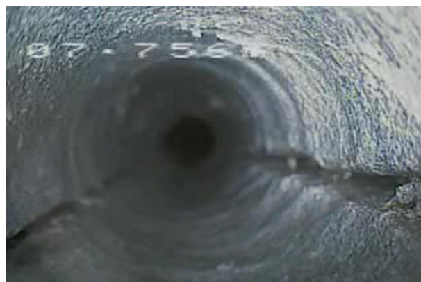
Figure 14. Borehole 5# image at the central position.
