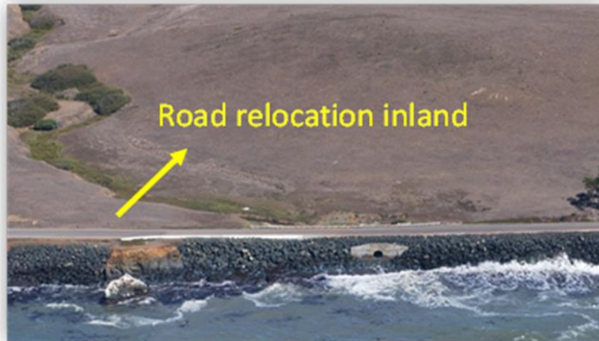
Figure 22. Photo depicting planned retreat for major public infrastructure. The Piedras Blancas Highway 1 Realignment will move nearly 3 miles (5km) of Highway 1 500 ft (152 m) inland. (Source: California Coastal Records Project )
