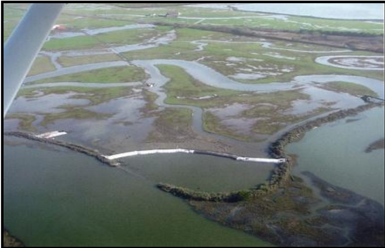
Figure 4: Existing Levee in North Humboldt Bay (Source: Water Structures, 2004)
