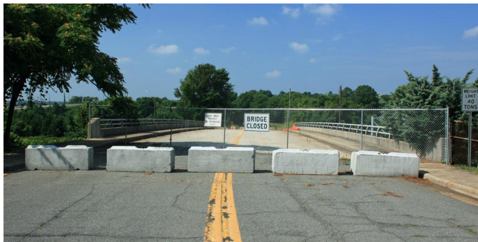
Figure 4.4. Greyhound Court Bridge, northeast approach.
