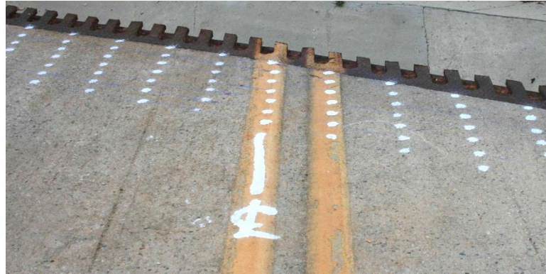
Figure 5.7. Painted SPA test points at the centerline.
