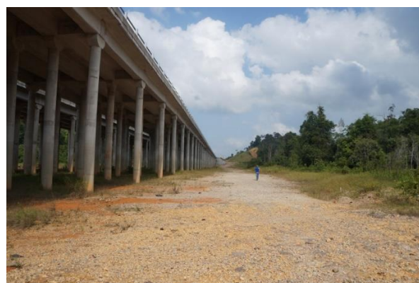
Fig. 1: A photo of post-construction at East Coast Highway Underpass (Source: PERHILITAN, 2018)
