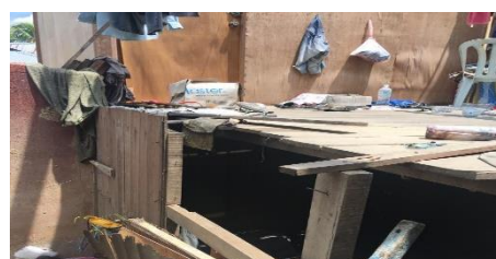
Fig. 7. (a) Roofing damage and transported a distance away due to failure of poor connection and use of lightweight zinc materials creating higher net uplift forces (b) Loss of wall frame due to poor connections between wood and brick wall (Source: Field survey reports by APM)
