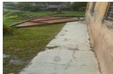
Fig. 7. (a) Roofing damage and transported a distance away due to failure of poor connection and use of lightweight zinc materials creating higher net uplift forces (b) Loss of wall frame due to poor connections between wood and brick wall (Source: Field survey reports by APM)
