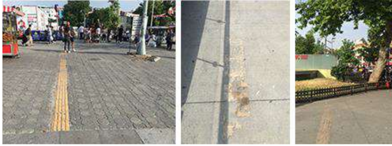
Fig.13.Guide surfaces for visually impaired people in Kadıköy Square (Source: Kutsal Göllü, Canbay Türkyılmaz, 2018)
