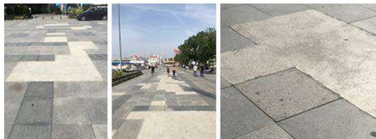
Fig.11. Concrete floor renovations in Kadıköy Square (Source: Kutsal Göllü, Canbay Türkyılmaz, 2018)
