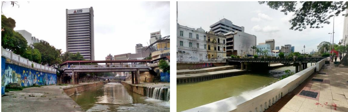
Fig. 4. Bridge conditions at Precinct 7, ROL Project Sources: Google Street View (2014)
