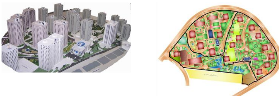
Fig 3. Hormozan residential complex
