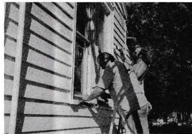
4) Custom work by the boys. Curt trims out window; Snowball replaces rotten window casement.
