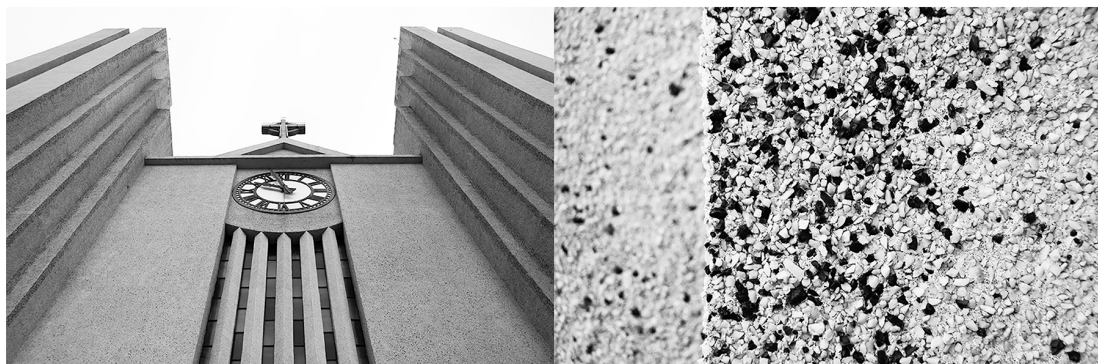
Figure 7. Steining on the church of Akureyri. Detail on the right. Photos by Sofia Nannini.
