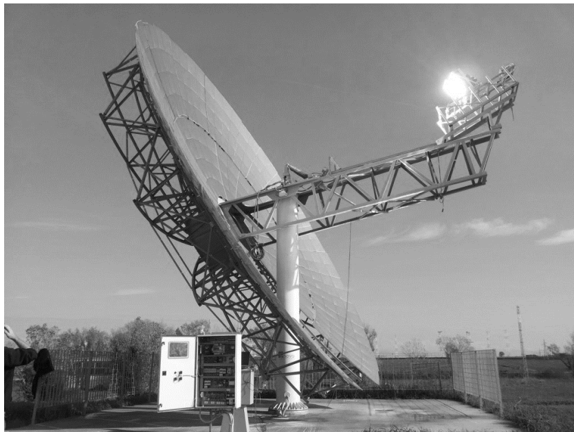
Figure 3. OMSoP project dish CSP system. Source: https://etn.global/
