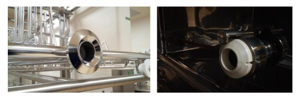
Fig. 3. 1: Coupling mechanism: Left: Female fitting on rack, right: male fitting in washer.
