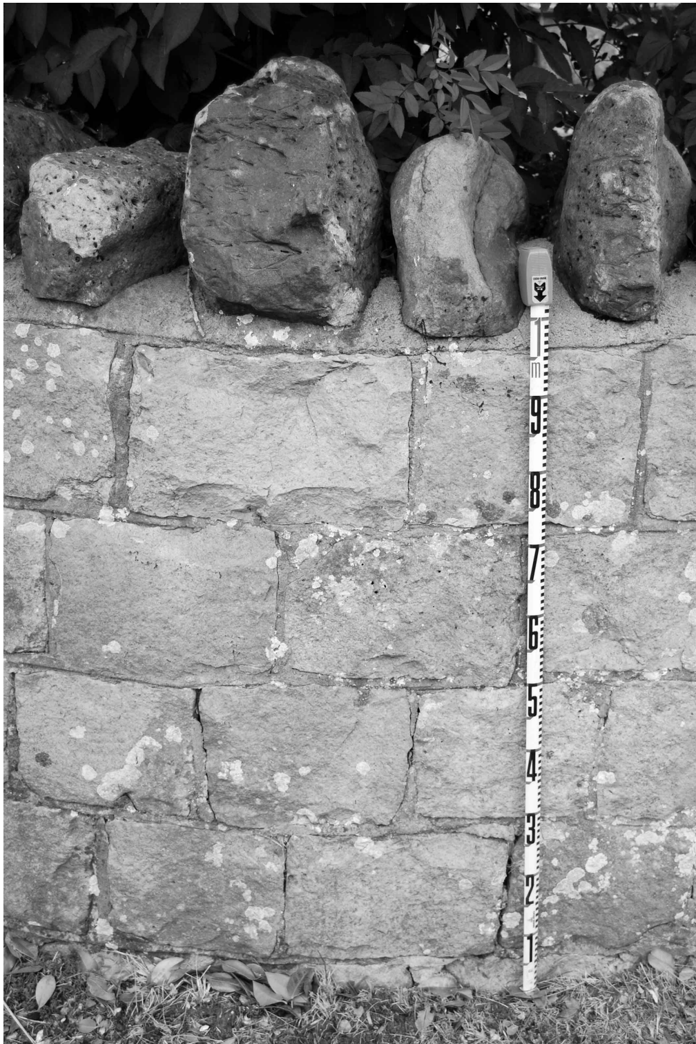
Figure 2 The churchyard wall, Fyfield (Wiltshire), constructed from cut blocks of saccharoid sarsen, capped with quartzitic sarsen nodules (© author).
