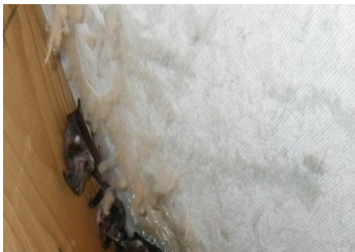
Figure 14. ‘Fluffing’ of a BRM surface four months after being fitted in a bat roost (Sample B)
