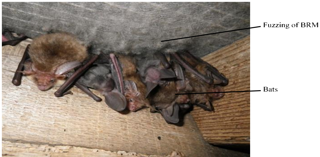
Figure 4. Example of fuzzing on a nonwoven membrane within a bat colony (Courtesy of John Martin, Cumbria, UK)
