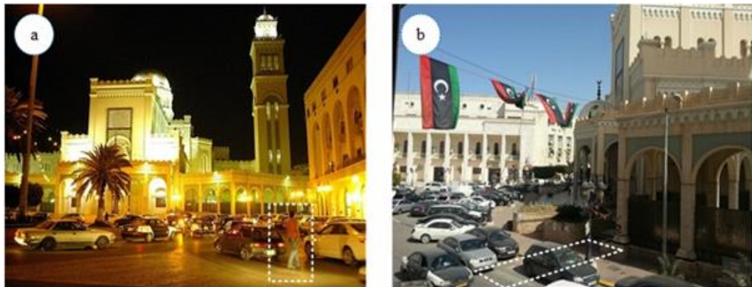
Figure 8-20 Lack of traffic lights and pedestrian crosswalk
