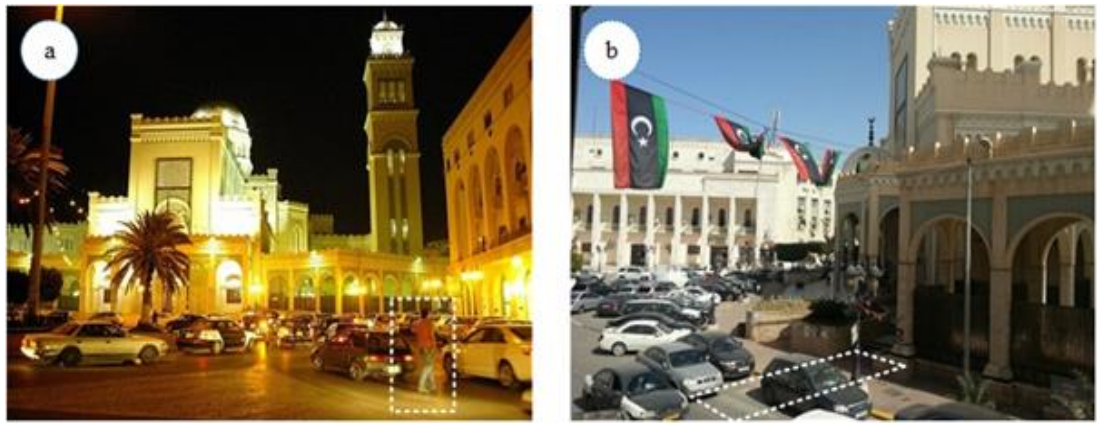
Figure 8-16 Lack of pedestrian access
