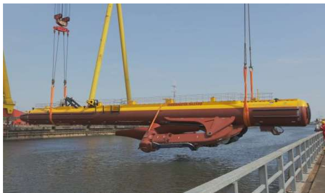
Figure 1: Scotrenewables Tidal Power's SR2000 tidal current turbine being deployed
