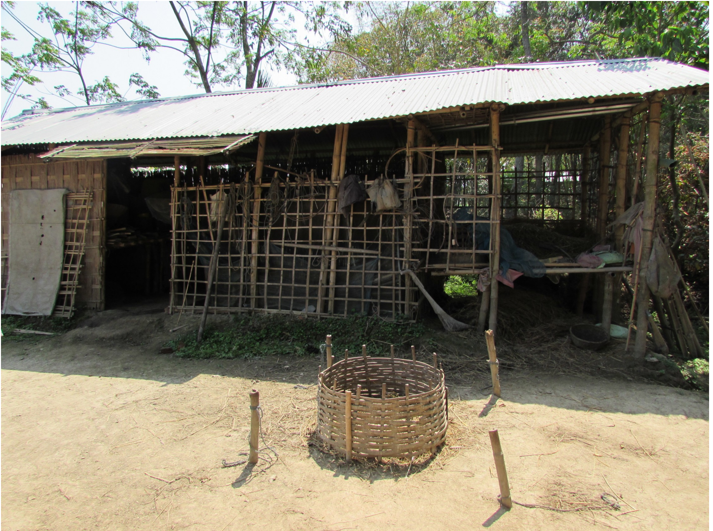
Fig 2. Typical livestock accommodation. Built from bamboo with a corrugated steel roof for protection from the rain, this structure is not entirely secure against large predators such as tigers. The central area of the accommodation might be used for cattle and goats, or goats could be accommodated elsewhere in a raised structure. The mud floor of the accommodation is slightly raised for drainage, important if hygienic conditions are to be maintained. The right section is a store for conserved fodder, mostly rice straw, the raised left section is a store for firewood. Poultry will also share this accommodation, and some farming implements and fishing tools stored inside. Note the ring feeder for fodder with four tether points in front of the structure.
