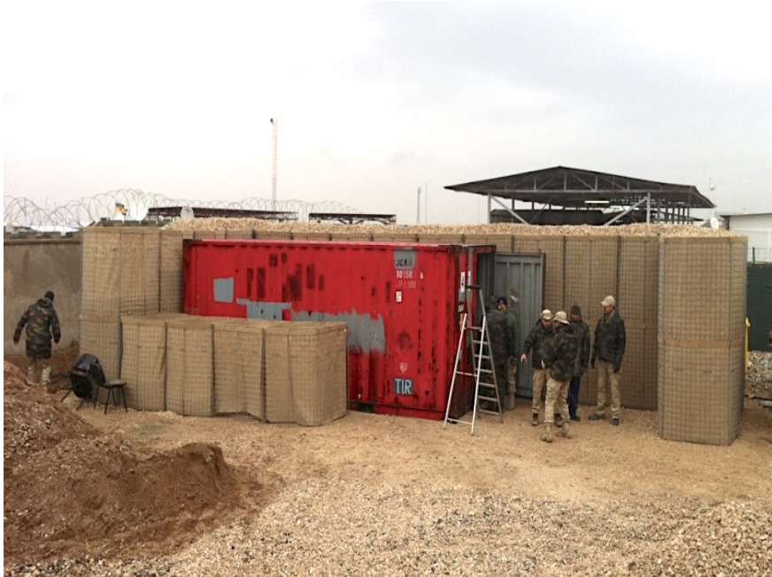
Fig. 1 Hesco-Bastion survival shelter configuration during construction [1].
