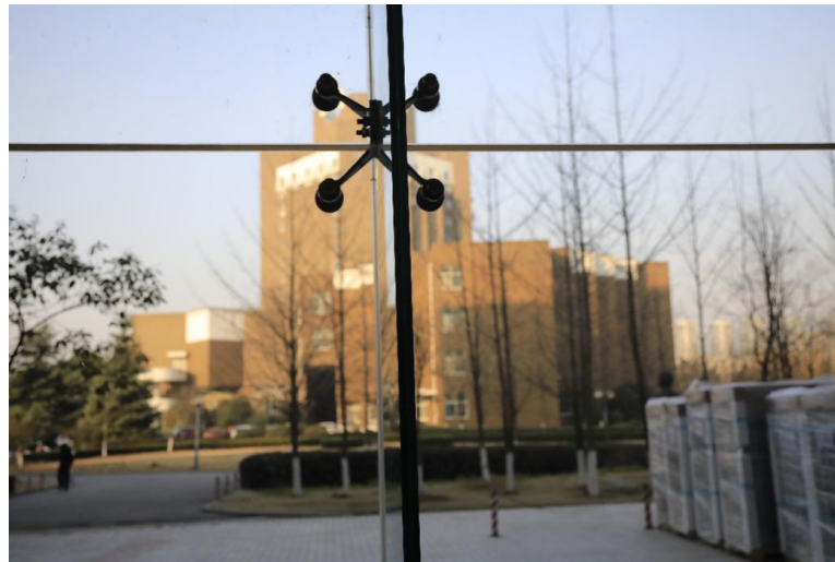
89 90 Fig. 1. Point-supported glass curtain wall, USTC campus, Hefei.
