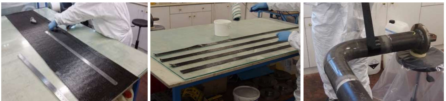
Fig. 2: Implementation of the CFRP patch on the pipe elbow.
