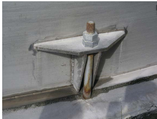
Figure 4: Typical anchoring in liquid storage tanks.
