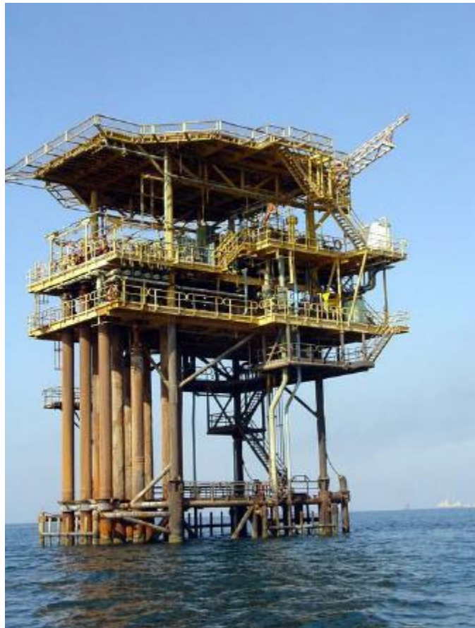
Figure 1 – Typical Ageing WHPT in Shallow Water Fields [1]
