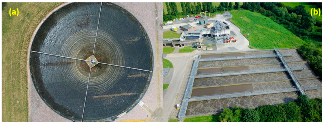
Figure 1. (a) Example of trickling filter and (b) example of activated sludge within two independent wastewater treatment plants.
