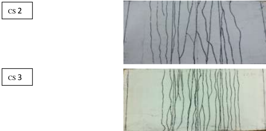
Figure 6 Failure patterns of ferrocement slabs
