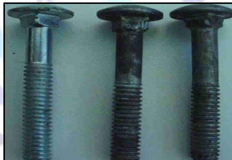
Fig. 9 - Corroded cadmium-coated steel bolts
