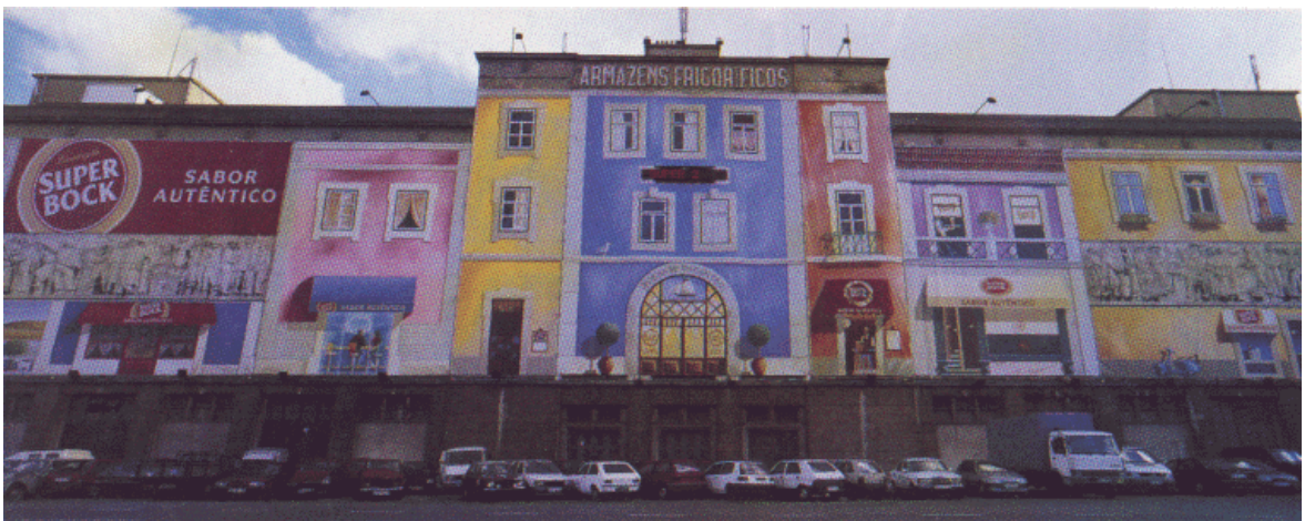
2. Facade of a warehouse covered with large-scale advertising. This building has an excellent visibility from the busy avenue that stretches along the riverside. Quay of Alcântara – Lisbon, November 2000.
