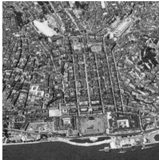
20. Aerial view of Baixa , Lisbon 1999. The construction work for a new subway station and a tunnel for the traffic passing by the water front are visible at Terreiro do Paço . Terreiro do Paço's water front will be free of traffic.
