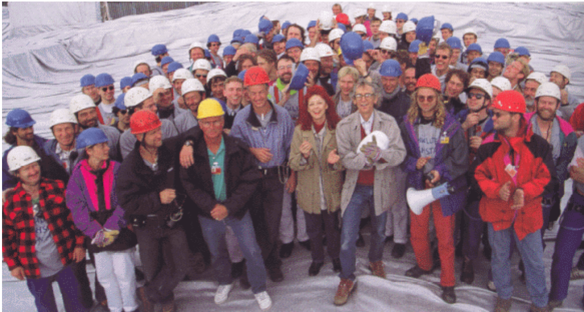
50. After the roof was fully covered, Jeanne-Claude and Christo joined the workers for a group photograph. June 1995.
