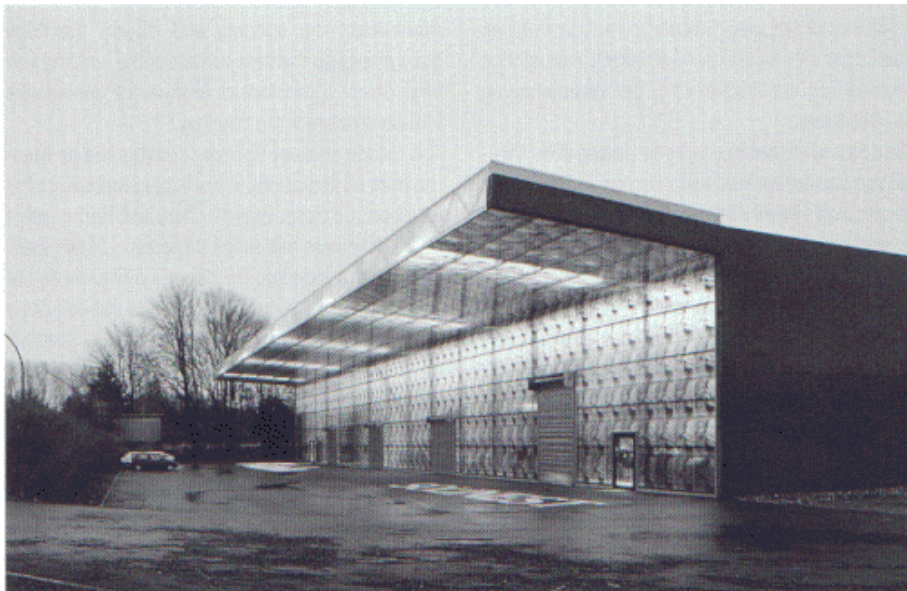
61. Herzog & de Meuron, "Ricola-Europe SA. production and storage building" Mulhouse-Brunstatt, France, project 1992, realization 1993, ground view with nightlight conditions. The polycarbonate facade.
