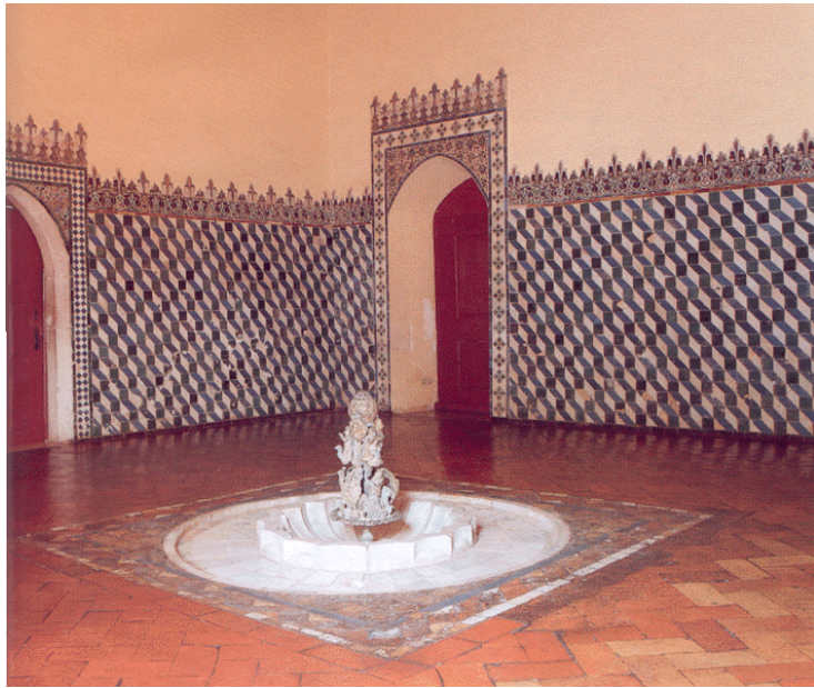
23. Sala dos Árabes, Palácio de Sintra, sixteenth century, zigzag composition with fat glazed tiles combined with low relief glazed tiles on the frieze.
