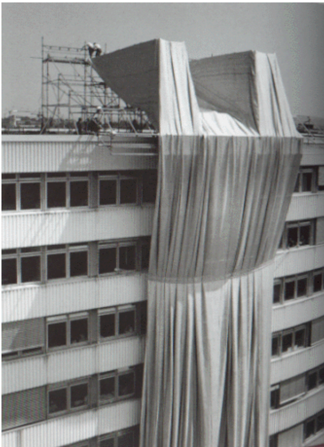
47. Test wrapping. The IPL team first constructed a framework of steel pipes, creating a three-dimensional form that corresponded to the angular configuration of the Reichstag's roof. Then they inflated a large air cushion, designed to fill out the space between the two "ears." The use of inflated air cushions provided a flat top surface for workers to unroll the fabric over the edge of the roof.
