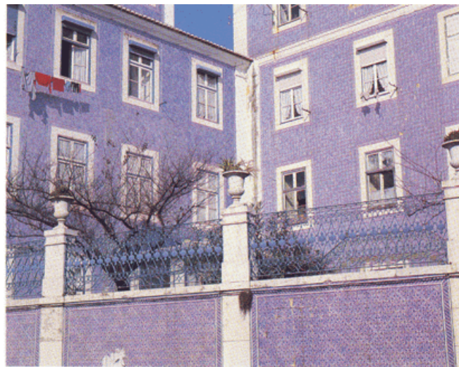
36. Facade with industrial tiles, late nineteenth / early twentieth century, building located at Calçada dos Marqueses de Abrantes, Lisbon.
