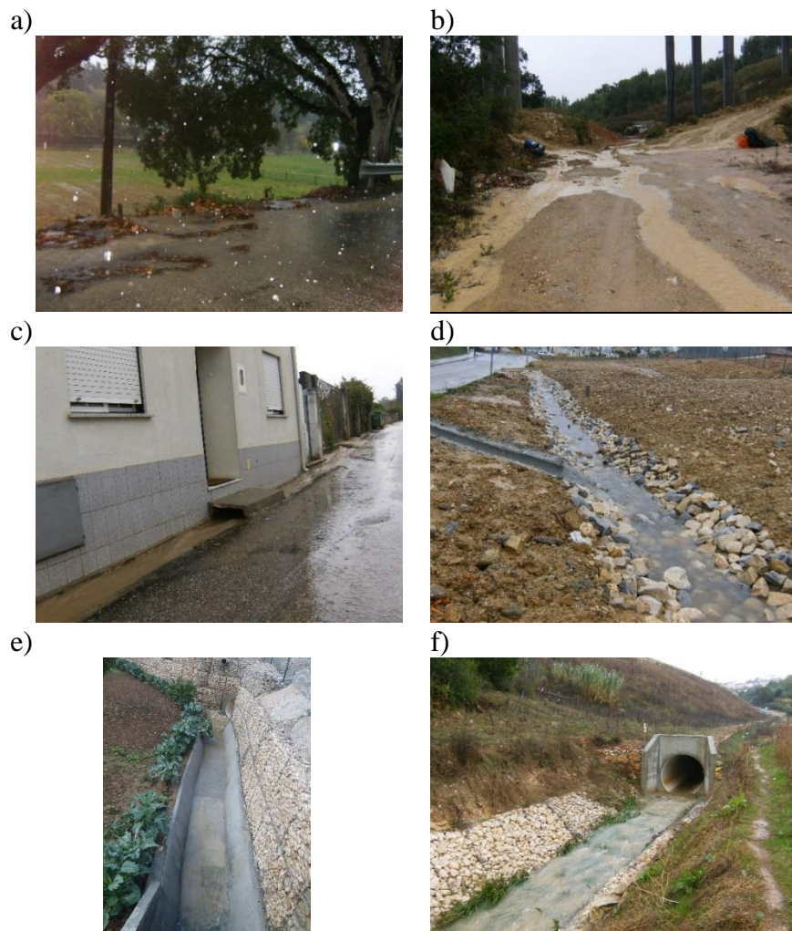
Figure 5.31 - Contrasting stormwater management strategies: a) overland flow runs freely to downslope agricultural or b) woodland soils; c) storm drainage systems collect and deliver overland flow into the stream network, downslope section of ESAC catchment and d) downslope Drabl ; and e) stream channelization within downstream Porto Bordalo and f) Drabl .
