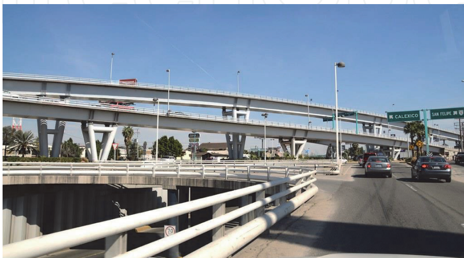
Figure 8. Mexicali bridges, road distributor [9].
