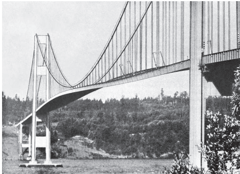
Figure 9. Tacoma narrows suspension bridge, under aerodynamic vibrations [10].
