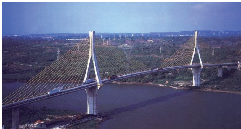
Figure 10. Coatzacoalcos II cable-stayed bridge overview [11].
