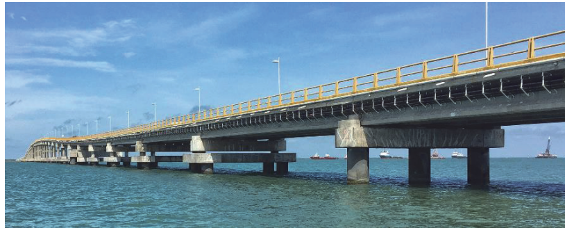
Figure 7. Bridge of pre-stressed concrete Girders el Zacatal, México [7].
