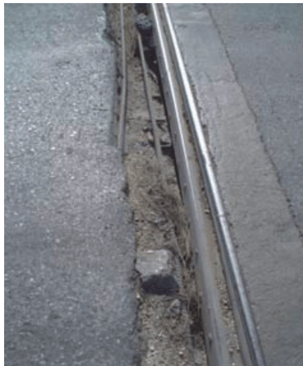
Figure 21. Bridge concrete construction joint damaged [20].
