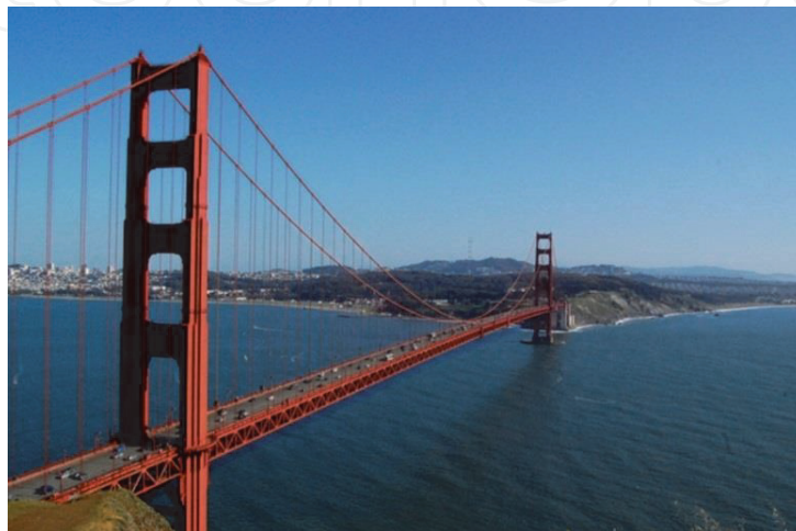
Figure 6. Golden Gate suspended bridge, San Francisco, U.S.A. [6].
