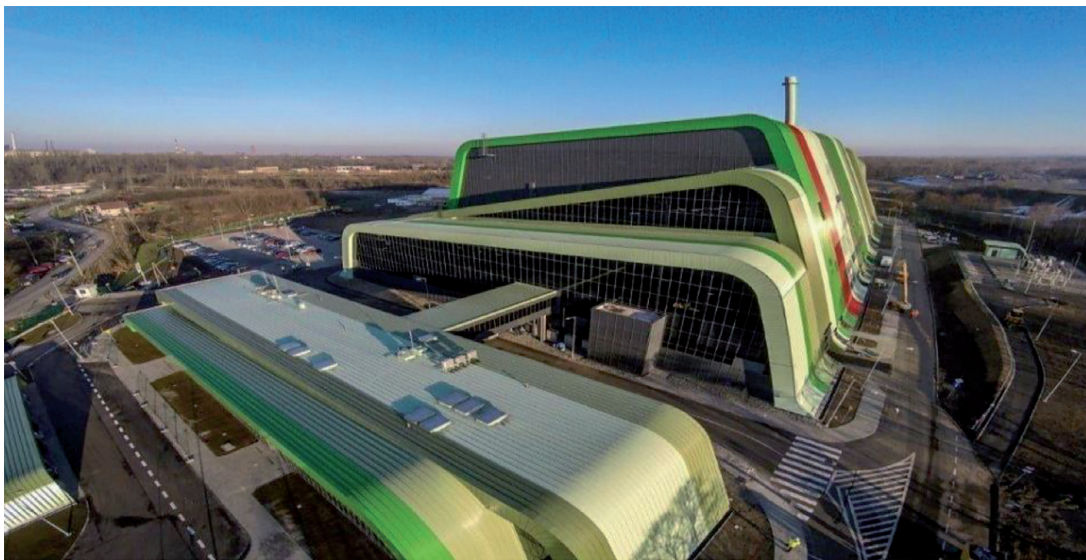
Figure 12. The thermal waste treatment plant in Krakow [31].
